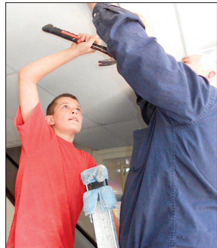
Garrett Thompson nails weather-stripping around Church front doors.
